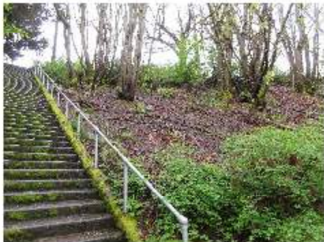
View looking west towards 31 st Avenue South at bottom of southwest staircase.
