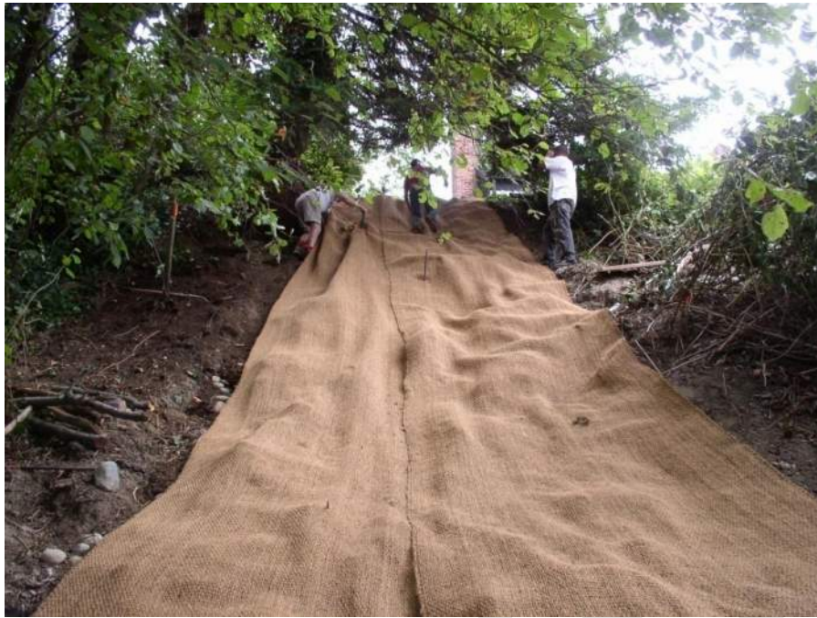
1. Coir fiber erosion blanket placed over bare soil after a slide event.
