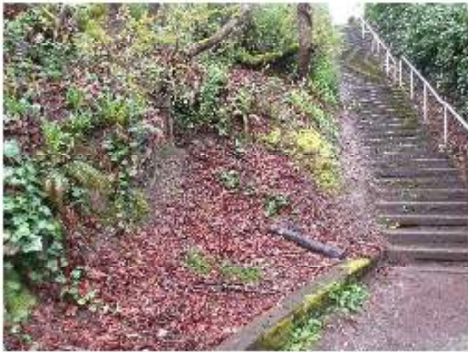
Wide angle of southern side of steep upper slope area to the left of the southwest staircase. Invasive English ivy noted.
