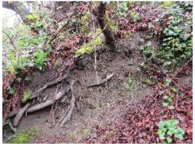
Exposed roots along the southern side of the steep upper slope area to the left of the southwest staircase.
