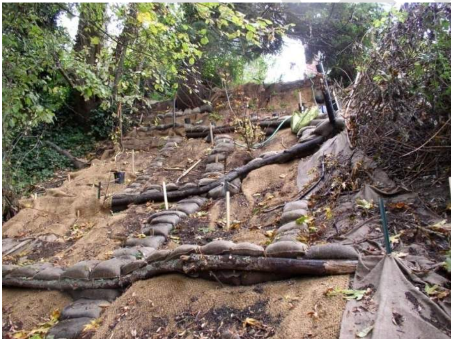
2. The same slope with the addition of sand bags and new plant installation. Large woody debris was added over much of the coir blanket. Natural leaf fall from adjacent trees covered the surface over the following years.
